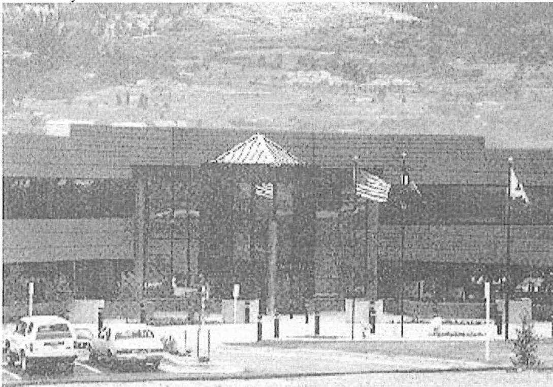
The Colorado Springs headquarters building looking southwest toward the foothills.
